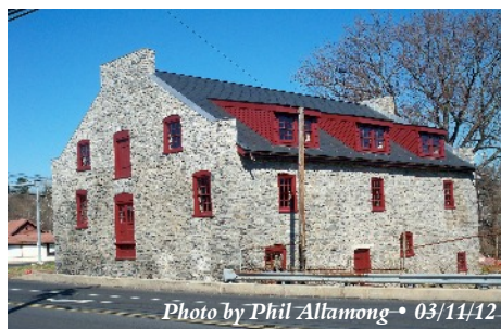
Photo by Phil Allamong • 03/11/12 This is how the Mill looks today after being refurbished with stone work and new doors and windows (as viewed from Stone Mill Rd.)
